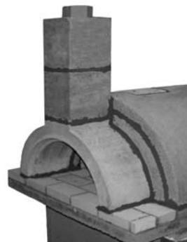
Completed Installation, Ready for Finish Application
