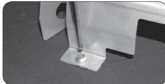
Fig. 15-2 Fastening hammer screws
