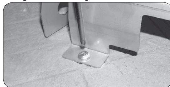
Fig. 15-2 Fastening hammer screws
