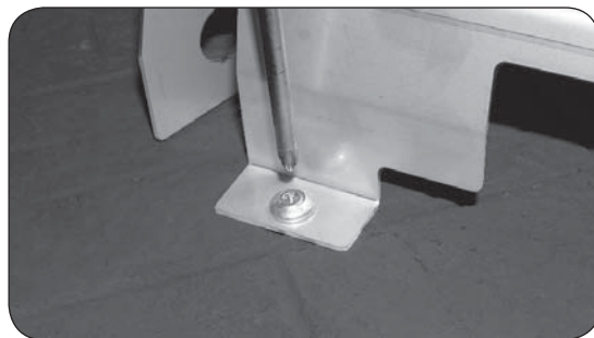
Fig. 10-2 Fastening hammer screws
