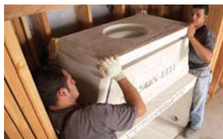
4. Finishing with the dome top
