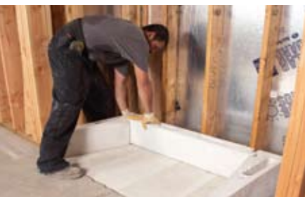
1. Installing base and first course
