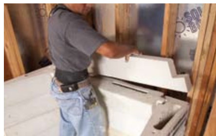
2. Starting the smoke chamber
