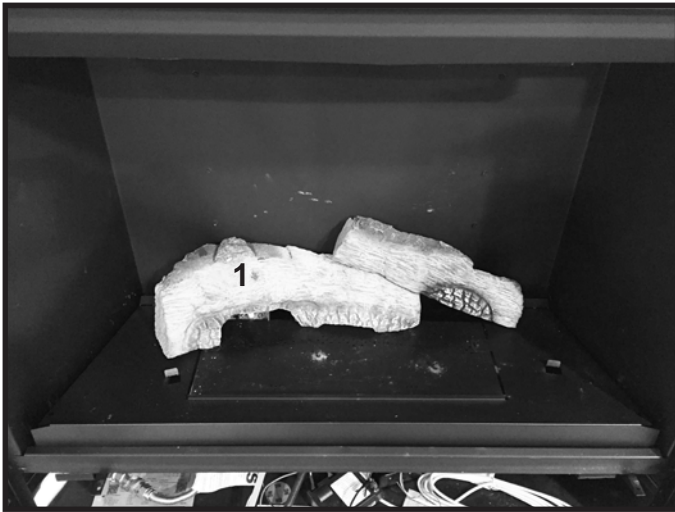
Figure 4. Install Left Rear Base Log
