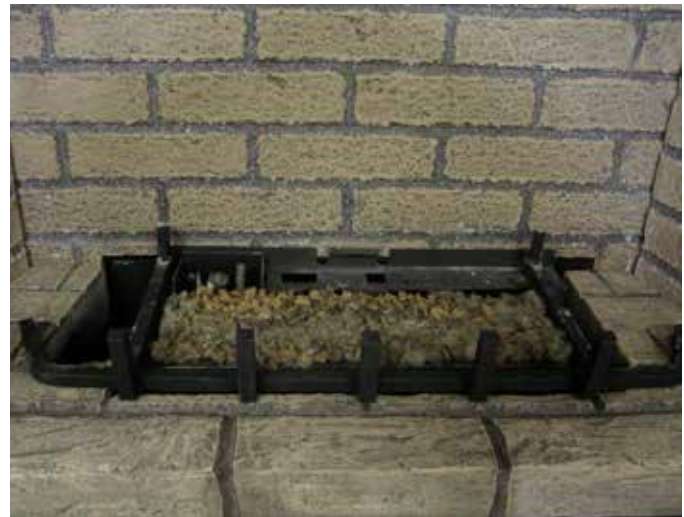
Figure 39 - Placement of Rock Wool on Burner
