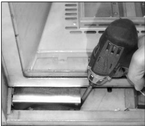
Power Vent Control Module Mounted inside fireplace.
