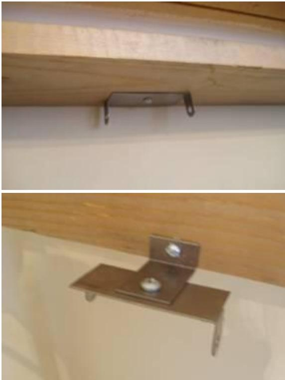
Attach the center bracket (or the combined brackets, for arched fireplaces) to the lintel using either a lag bolt for your masonry fireplace or a metal screw for your metal firebox.
