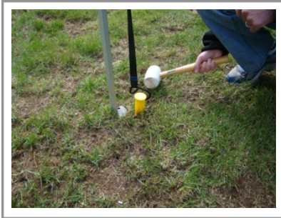
2) Hammer Stake into ground next to leg
