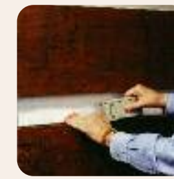
2. Tape the entire joint using polyester tape.
