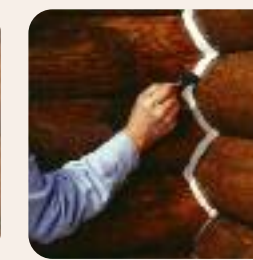
4. Tool to ensure a tight seal.
