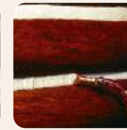
3. Gun Log Jam over the backer rod.
