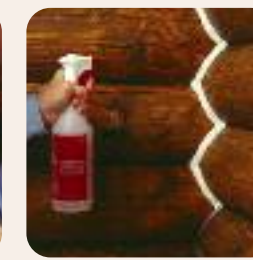
3. Lightly mist the Log Jam as needed.
