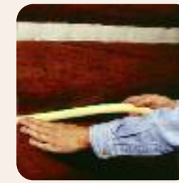
2. Or, install backer rod into caulk well of clean, stained logs.
