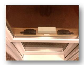
This is an example of a PROPER installation. In this application you can successfully utilize loop1 (the shock processor) and loop 2 (the internal reed switch)
