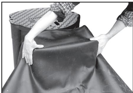
Position pond liner over the Skimmerfilter™ mouth and hold it in place. Smooth liner free of wrinkles and folds. Wipe clean.
