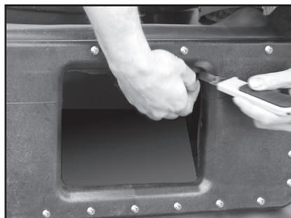
After the faceplate is properly tightened down, use a knife to trim the liner inside the mouth of the Skimmerfilter.™
