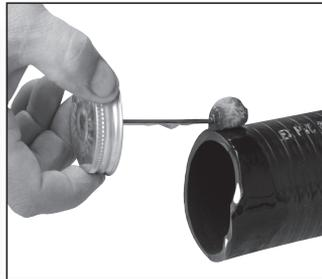
Apply the purple primer on the inside of the 90° elbow and on the outside of the SAVIO Aqua Flex PVC™. Repeat, using wet weld glue.
