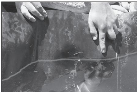
With the pond full, mark position of water level on the liner at the Skimmerfilter™ location. Drain pond partially 8"-10" inches before proceeding.
