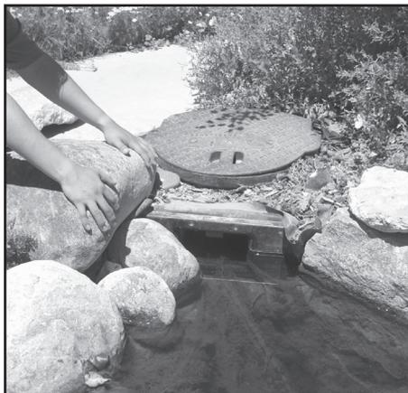
To hide the Skimmerfilter™ from view, extend coping shelf rockwork up to both sides of the Skimmerfilter™ opening.
