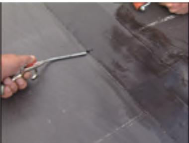
**Step 7-** Using a compressed air source, test all bonded seams using a minimum 50 p.s.i. (344.74 kPa) air supply directed through a 0.1875" (0.48 cm) nozzle held within 2.00" (5.08 cm) of the seam edge.
