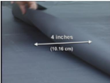
**Step 2-** Overlap the adjacent PondGard panels by a minimum of 4.00" (10.16 cm). Allow the PondGard panels to relax for 15 minutes.
