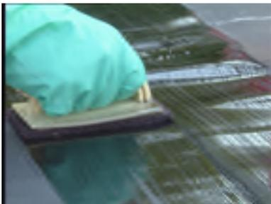
**Step 3-** Using a scrubber pad and holder; apply the QuickPrime™ Plus Primer to the top surfaces of the adjacent PondGard panels covering a minimum of 4.00" (10.16 cm) on both sides of the overlap edge.
