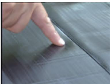
**Step 4-** Test the primer flash-off by touching the primed area with your finger and pushing forward at an angle. The primer should not string as your finger is moved up and away.
