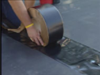
**Step 5-** Install the QuickSeam Cover Strip by using both thumbs in the core and rolling the tape away from your body. As you move forward, peel away the release paper and place it under your knee.
