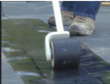
**Step 6-** Using either a hand or stand-up roller; roll the seam longitudinally and across the seam in overlapping sections to mate the seam together.
