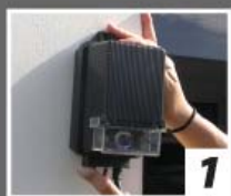
1 Mount/ position outdoor transformer
