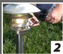
2 Route low voltage cable
