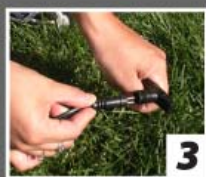
3 Connect fixtures to Quick Connect Cable
