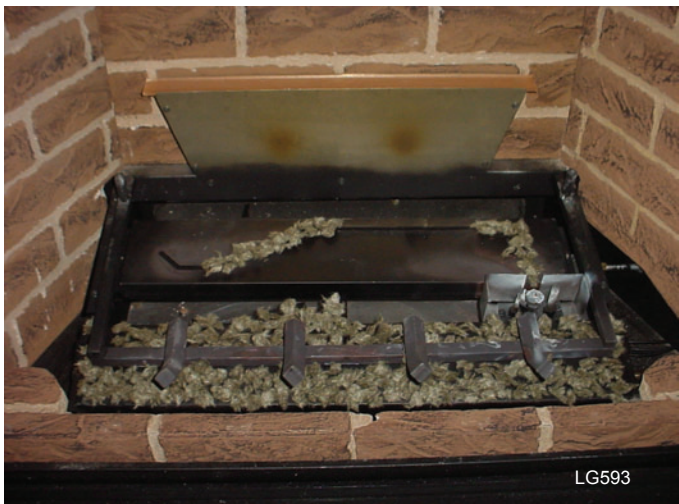
Burner Grate Assembly
