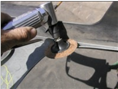
Picture #13: Grind the left over plastic nubs smooth.
