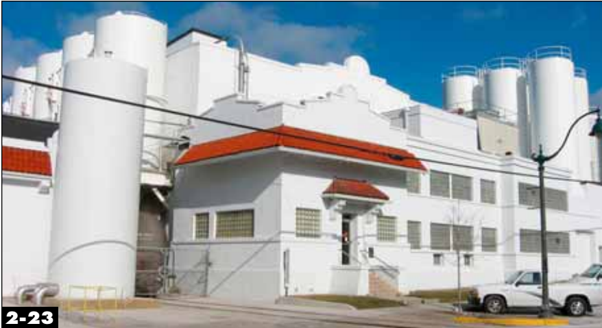
The modern Gehl Cheese plant in Germantown, Wis., receives sugar and soybean oil in tank cars. Bob Gallegos
