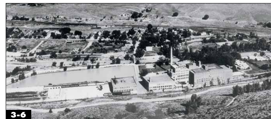
3-6 The Coors brewery in Golden, Colo., was served by multiple tracks from a curved spur off the main line at the top of the photo. In this early 1930s scene, several Coors billboard reefers are visible along with Pacific Fruit Express cars. Hol Wagner collection
