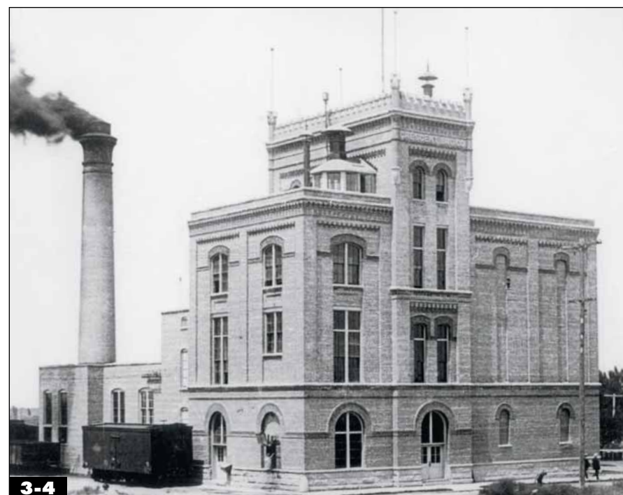
3-4 The Crescent Brewing Co., in Nampa, Idaho, was typical of small breweries in the early 1900s, featuring a multistory brick structure, tall smokestack, and rail siding. This view is from 1915. Jeff Wilson collection
