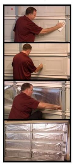
NOTE: There are eight (8) radiant barrier panels in the kit. Each panel is 4 feet in length. It is recommended that you use five (5) adhesive squares per panel. (5) per panel multiplied by eight (8) panels equal 40 adhesive squares necessary to complete the install. 48 squares are included in your kit to complete the installation.
