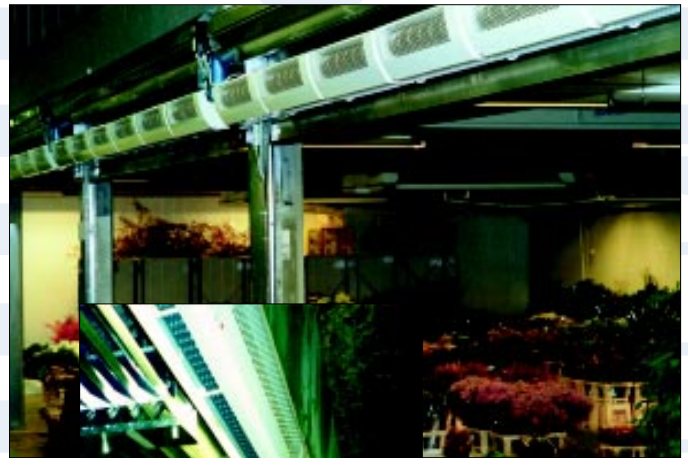
Fantech Air Curtains protect cold shops and refrigerated units – such as reach-in dairy and florist cases – from hot contaminated air, dust and insects.
