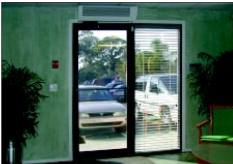
Fantech Air Curtains installed above doorways prevent hot air, dust and insects from entering air-conditioned rooms.
