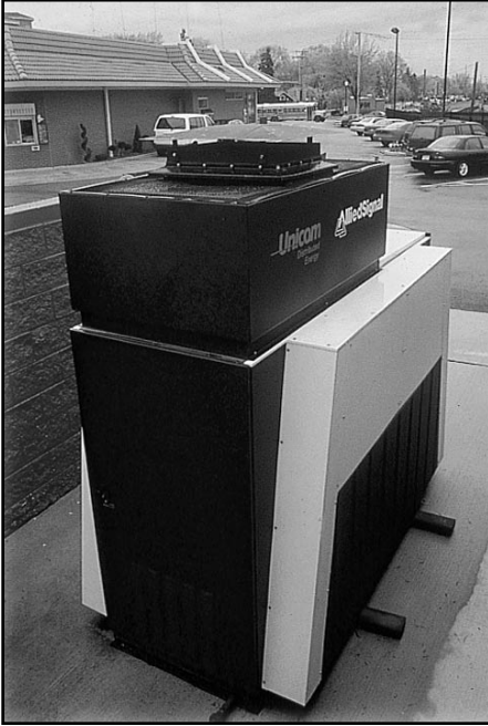
Fig. 1-6 Unicom Distributed Energy and Honeywell/Allied Signal Power Systems have demonstrated the Parallon 75 microturbine at an energy efficient McDonald's in Bensenville, IL.
