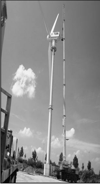
Fig. 1-2 Completion of a NedWind 500 kW wind turbine generator. The plant is expected to generate 2.6 million kWh annually, enough to meet the annual electricity demand of more than 800 households. Wind generation is particularly popular in rural areas, because it can allow farmers to generate additional income from grazing lands while still using the land for farming. The wind turbines use only a tiny fraction of the land they are sited on. Today's wind turbine models are far quieter than previous generations.
