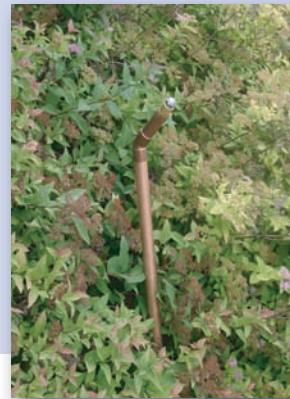
Nozzles (right) are placed at strategic locations based on landscaping and the structure of the home. The nozzles are connected to the pump/reservoir system (below).
