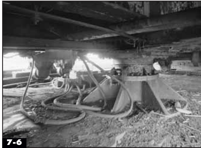
7-6 On a center-bearing bridge, the center bearing supports the entire weight of the bridge structure. The small wheels at the outside help balance the bridge as it pivots. Historic American Engineering Record; Wm. Barrett
