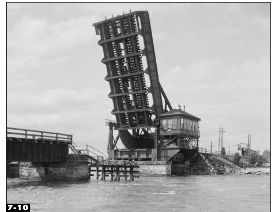
This double-track Scherzer rolling lift bridge was built on the New York, New Haven & Hartford near East Lime, Connecticut, in 1907. Historic American Engineering Record; Wm. Barrett
