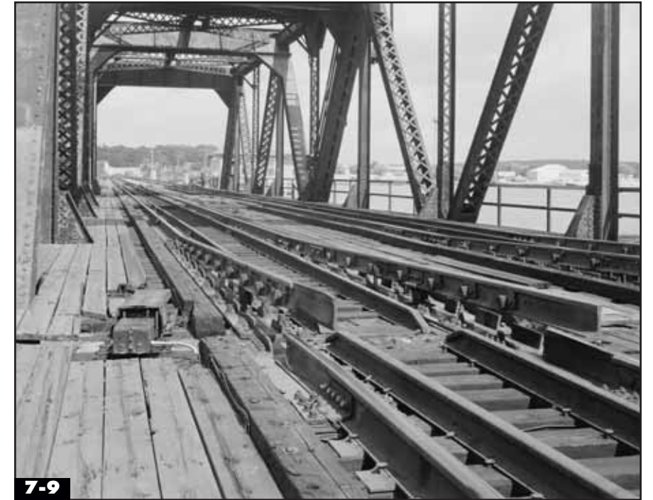
Rails, tapered at the ends, are hinged on the typical swing bridge. They are lowered to mate with the land-side rails once the bridge is closed and locked in position. Historic American Engineering Record; Wm. Barrett
