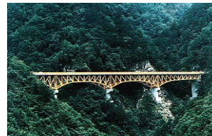
Mameyaki Bridge: 4 span continuous truss
